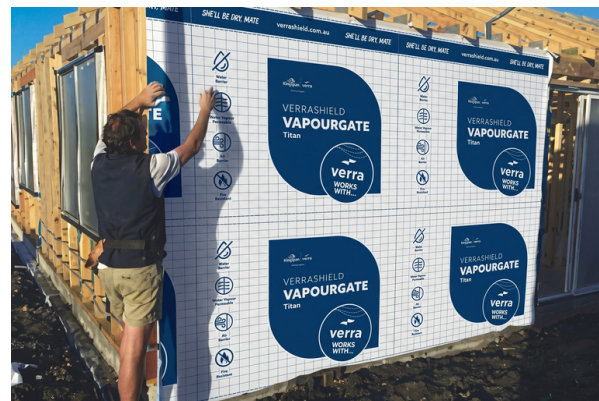
Figure 2. Fix Verra VerraShield VapourGate Titan securely to the frame.
