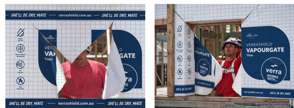
Figure 3. On arrival of doors and windows, cut the membrane at each opening on a 45° angle away from each corner. Pull the membrane flaps inside and fasten to the inside of frame.
